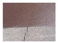
*Chip seal* -- This technique uses an asphalt emulsion (liquid oil) into which rock chips are rolled to restore the driving course. This surfacing treatment is not common in the city of Eugene but was used on Riverview Street in east Eugene, using a contracted Lane County road crew.
