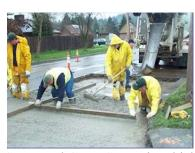
*Concrete panel replacement* – Failing panels of concrete roadway are removed, and new concrete panels are formed. This work typically is performed by Public Works Maintenance surface operations crews, usually during cooler and wetter weather that is not conducive to asphalt paving.
