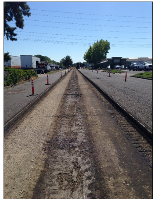
Pavement Removal on 5th Avenue
